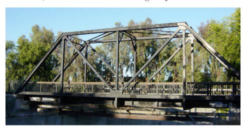
Figure 69 A simple truss
